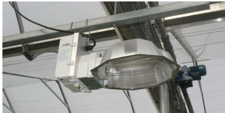
Figure 6. High Pressure Sodium lamp for supplemental lighting.
