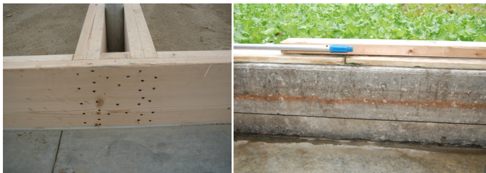
Figure 5. Edge of pond detail. The inside edges of two separate ponds made of wood and separated by structural members is shown on left. The right hand picture shows a concrete pond.
